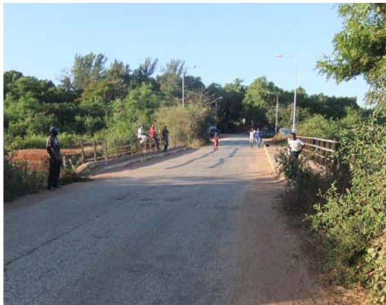
Bridge over Kotu Creek
